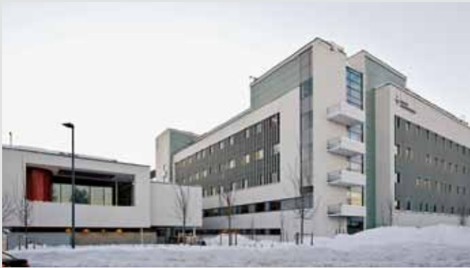
Akershus University Hospital, Akershus, Norwegen
