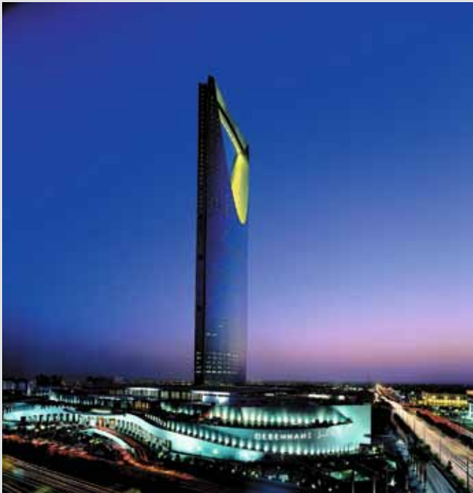
Kingdom Tower, Riyad, Saudi-Arabien
